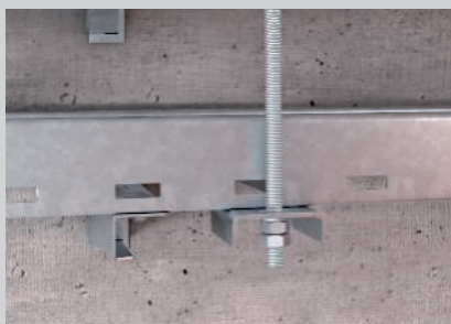
Fastening of the vertical threaded rod on the connection component.
