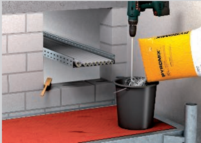
Stir the mortar with water until the desired consistency is reached.
