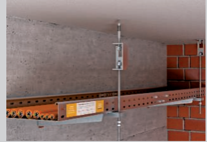
Ceiling fastening of the threaded rods with fire protection clamps.
