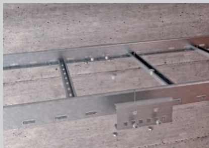
Mounting of the straight connectors using truss-head bolts.
