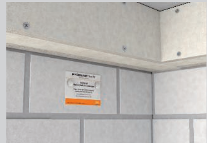
Labelling according to the VDE application rule.
