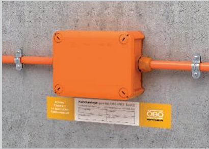
Fully installed FireBox with identification plate.
