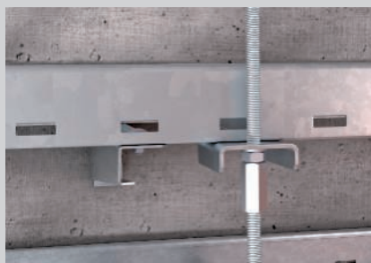
Threaded rod fastening on the cable ladder with multilayer arrangement.
