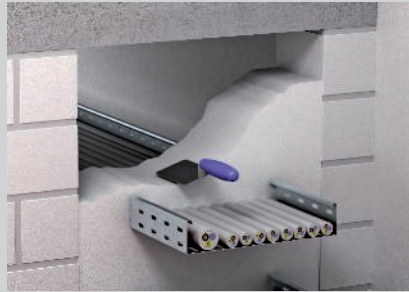
Apply mortar to the opening, use lining as necessary.
