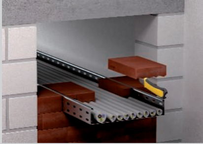
Mounting of the cut blocks.
