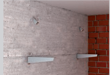
Mounting of the brackets and the sloping connection components on a wall.
