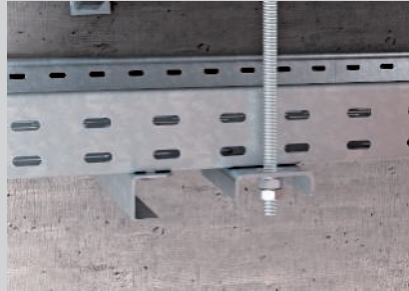
Fastening of the vertical threaded rod on the lowest cable tray.
