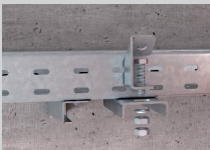
Fastening of the sloping connection component.
